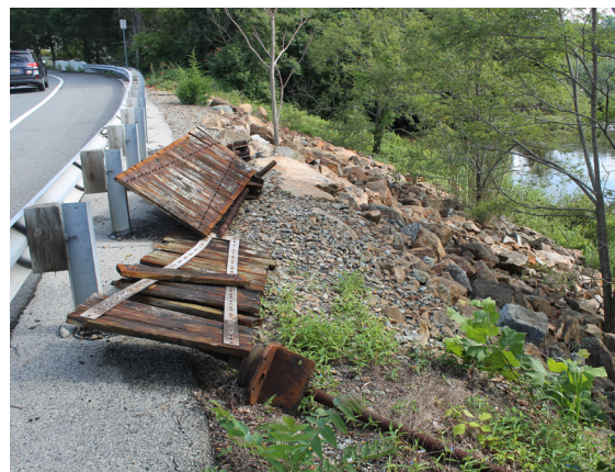
Detail of the original sluice gates and screw mechanism for Bridge 1-504 after having been removed and prior to repairs.
