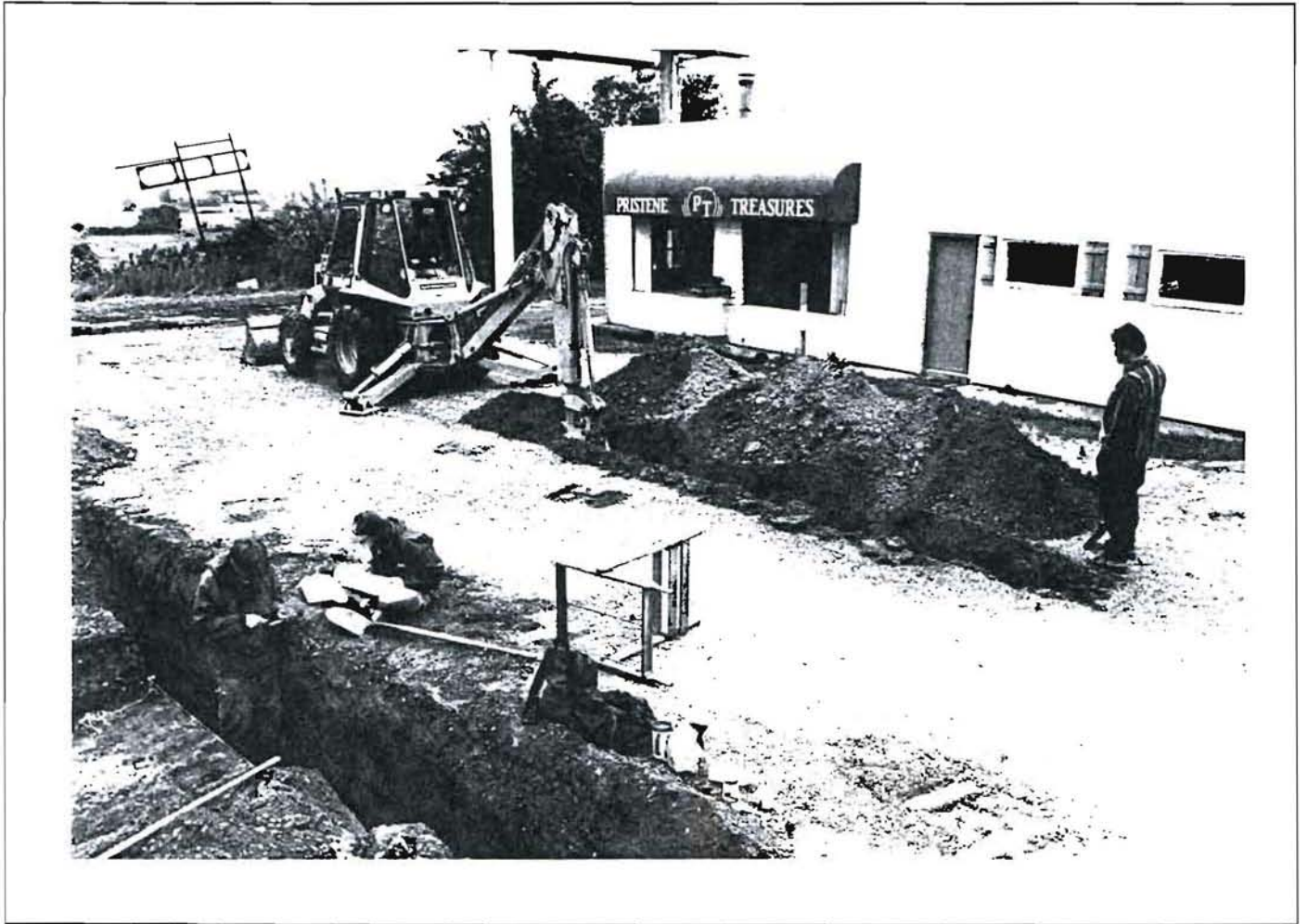
PLATE 19: Backhoe Trenching at the Weldin Store Site, 7NC-G-137
