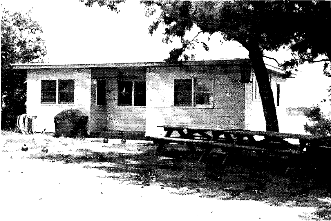
Plate 15. Ranger Residence (S-9804.001). Delaware Seashore State Park, North Indian River Inlet. West and south elevations toward northeast.
