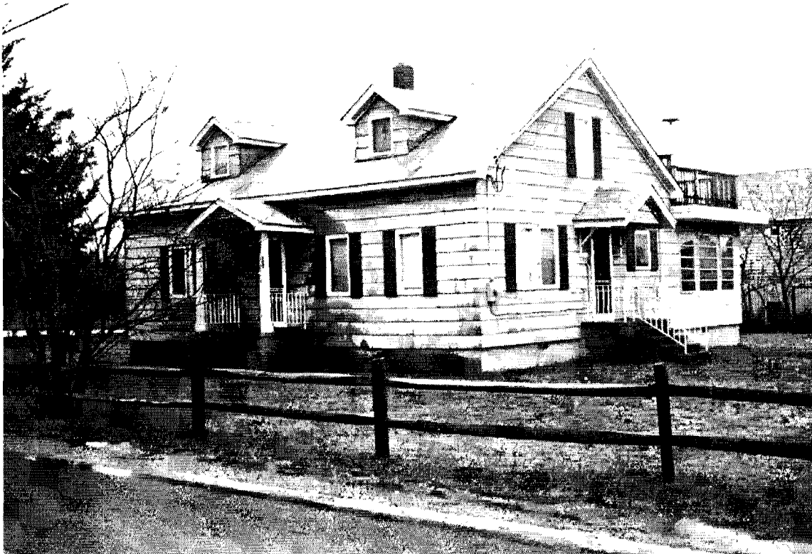
Plate 14. Summer cottage (S-2569). North of west end, Quillens Point Road. East and south elevations toward northwest.
