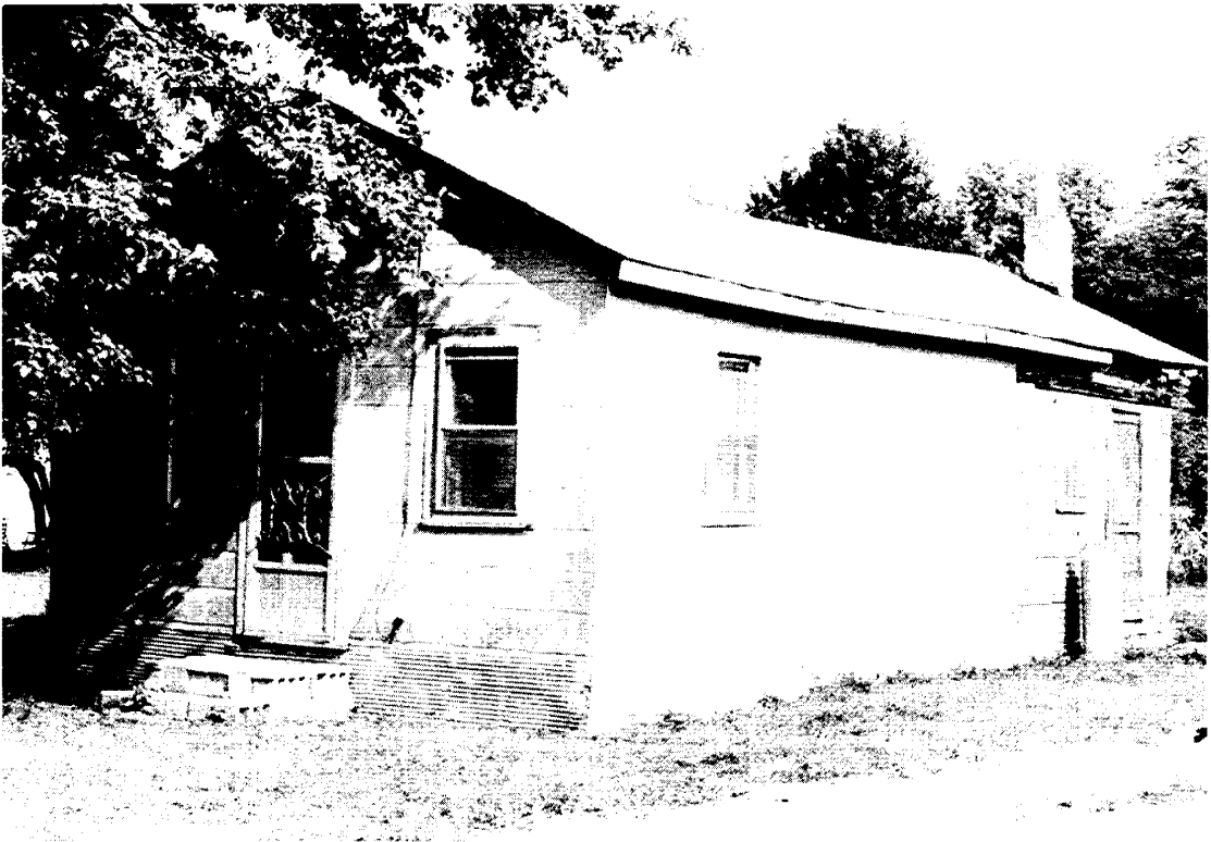
Plate 28. Jeroy Carter House (3-34-5-208), From the Northwest.
