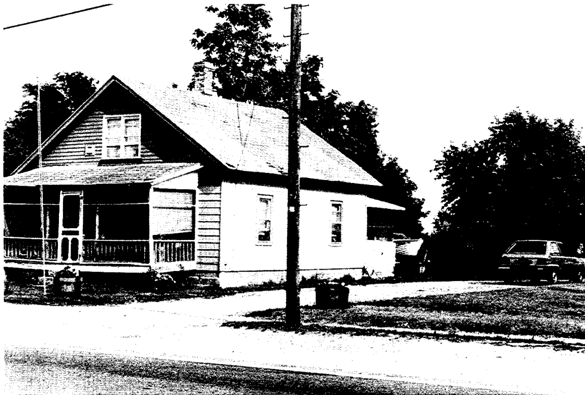
Plate 26. Irwin A. Coursey House (3-34-5-202), From the Northwest.
