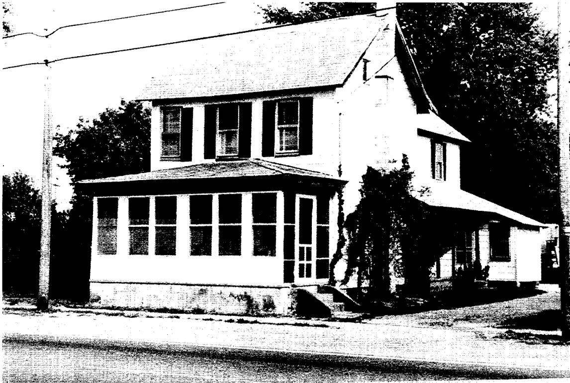
Plate 29. Jeroy Carter House (3-34-5-208.1), From the Northwest.
