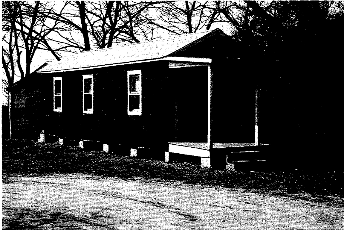
Plate 68. Francis-Anne Motel, Complex A (3-34-13.19-82), Rear Cottage, From the Northeast.
