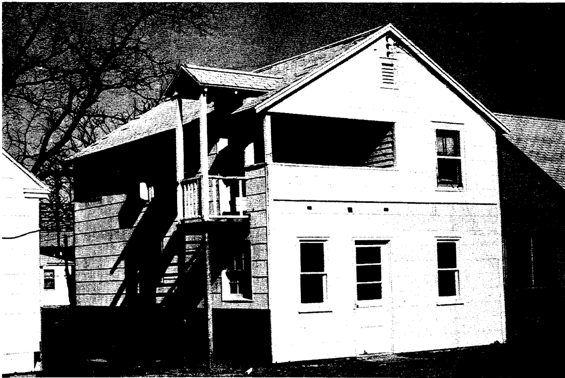
Plate 77. Francis-Anne Motel, Complex B (3-34-13.19-87), Cottage 8, From the South.
