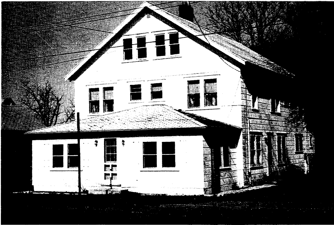
Plate 62. Francis-Anne Motel, Complex A (3-34-13.19-82), Large House, From the East.
