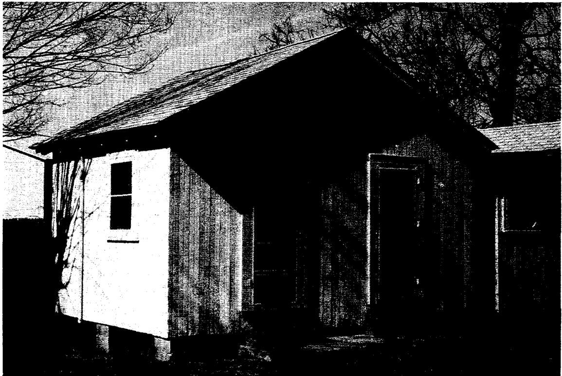
Plate 67. Francis-Anne Motel, Complex A (3-34-13.19-82), Cottage 4W, From the East.
