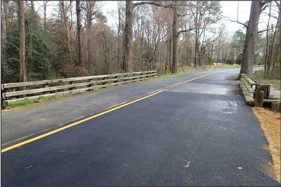
FIGURE 9: Recent Asphalt Patchwork on Rd. 72, Facing Northeast
