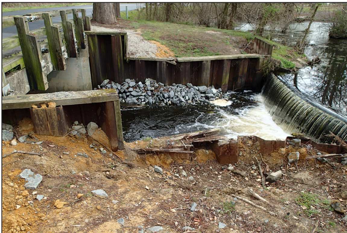
FIGURE 11: Damaged Cribbing and Recent Fill along Spillway, View Northeast
