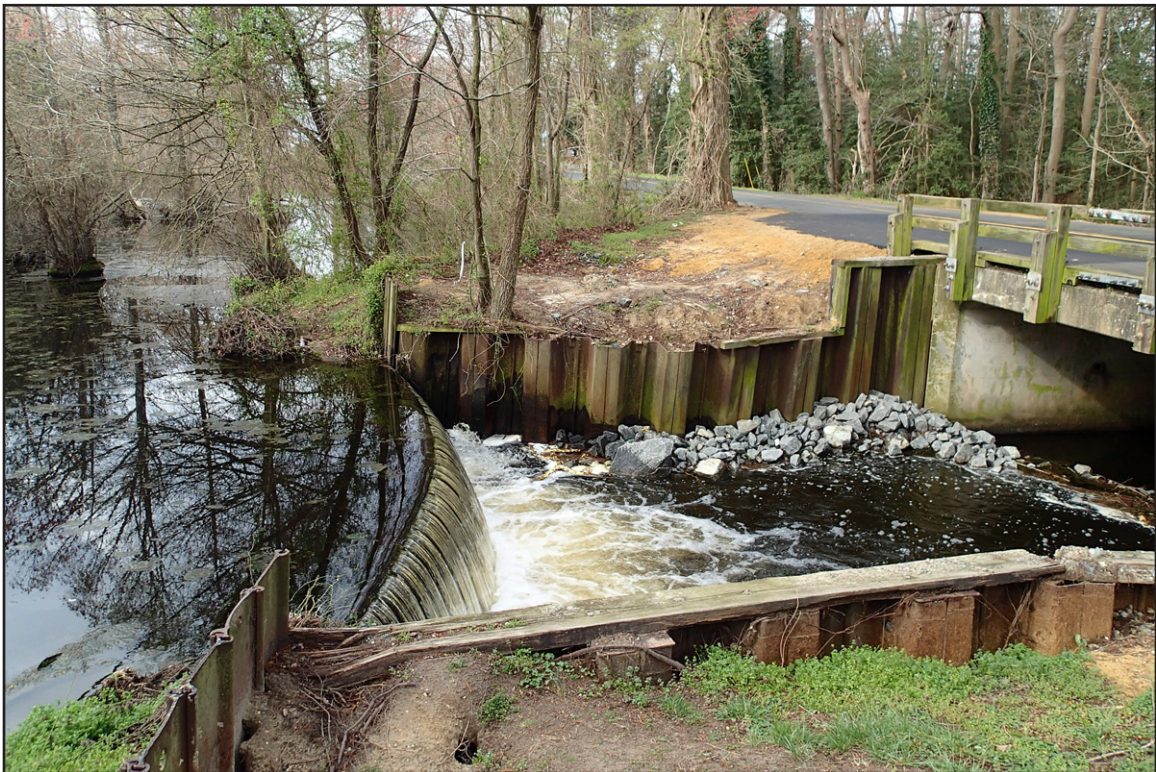
FIGURE 10: View of Weir and Spillway, Recent Fill and Asphalt Patchwork in Background, Facing Northeast
