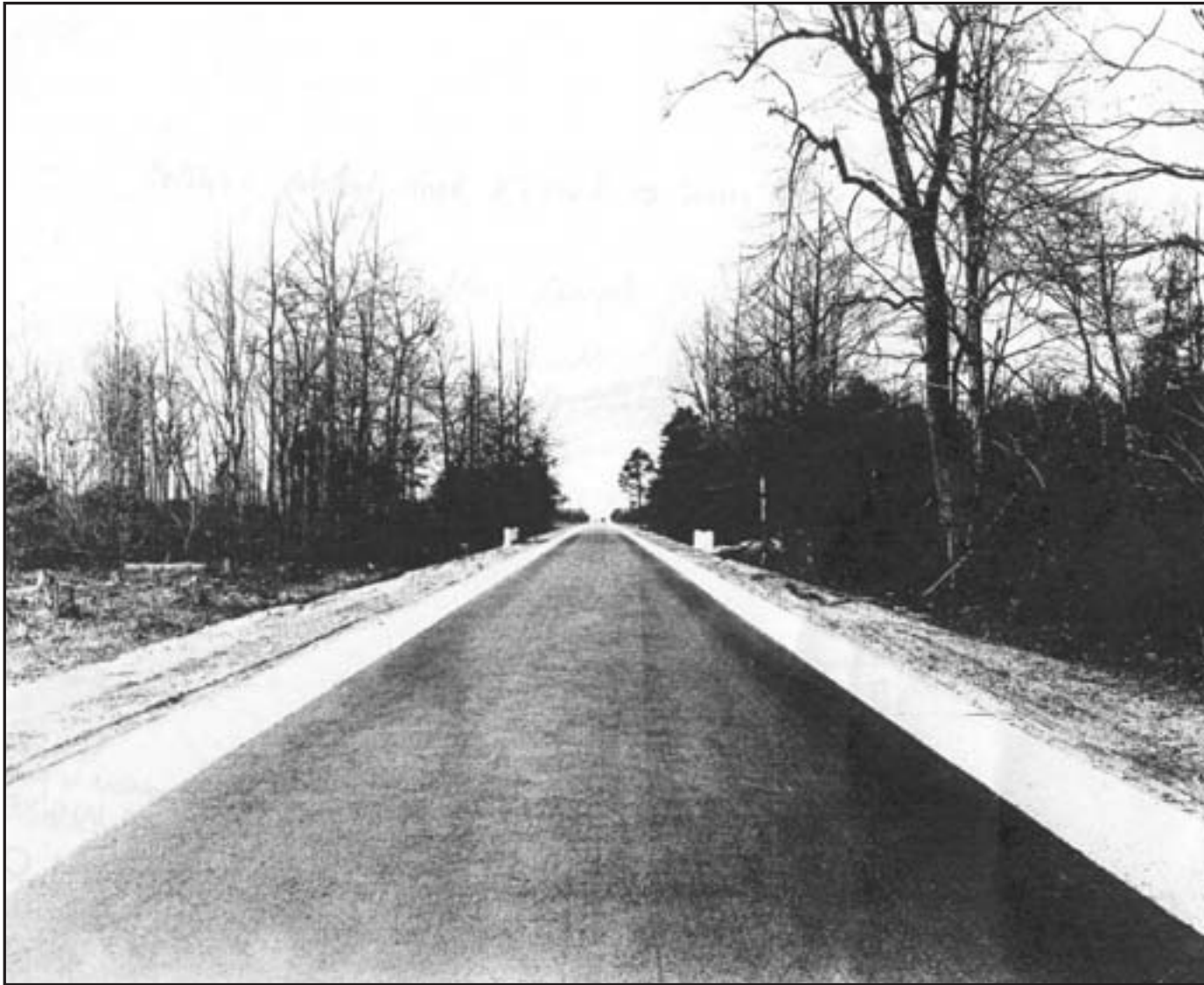
Figure 9. DuPont Highway, Sussex County. Updated photogrtaph showing concrete used to construct shoulders on highway. Delaware Public Archives RG 1540. Box 11, Folder 7. Photograph 894p.
