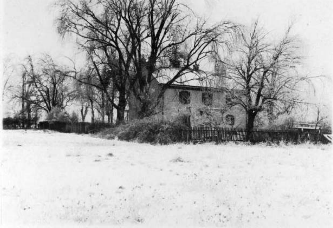
Photograph 19: Looking northeast at the rear of the main house. Note the chimney nearly centrally located where the two sections of the house were joined. The back yard is surrounded with a wooden picket fence.
