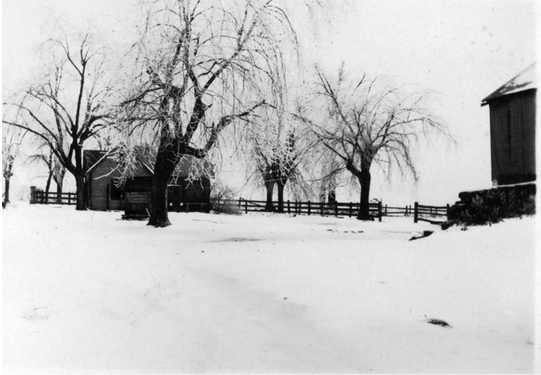
Photograph 22: Looking northeast at a corner of the stone wall to the barn ramp. Behind the ramp is the entrance to an equipment shed incorporated into the main block of the barn. The main house is to the left.
