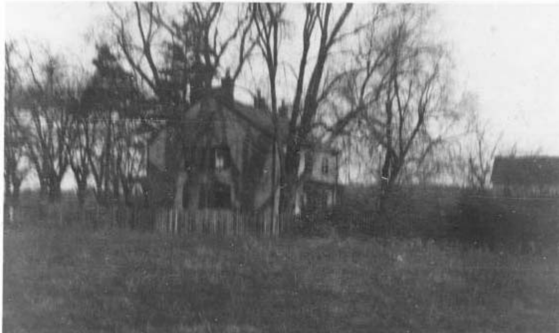
Photograph 18: Looking northeast at the west gable end of the main house showing the large gable end chimneys at that location.
