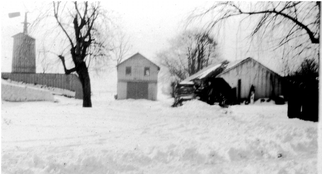
Photograph 23: Looking south at the frame, two-story, combination corn crib/wagon shed with board and batten siding. To the right is a frame equipment shed with an attached animal pen. To the left beside the barn ramp is a frame shed covering the cistern and topped with a frame water tank and windmill.
