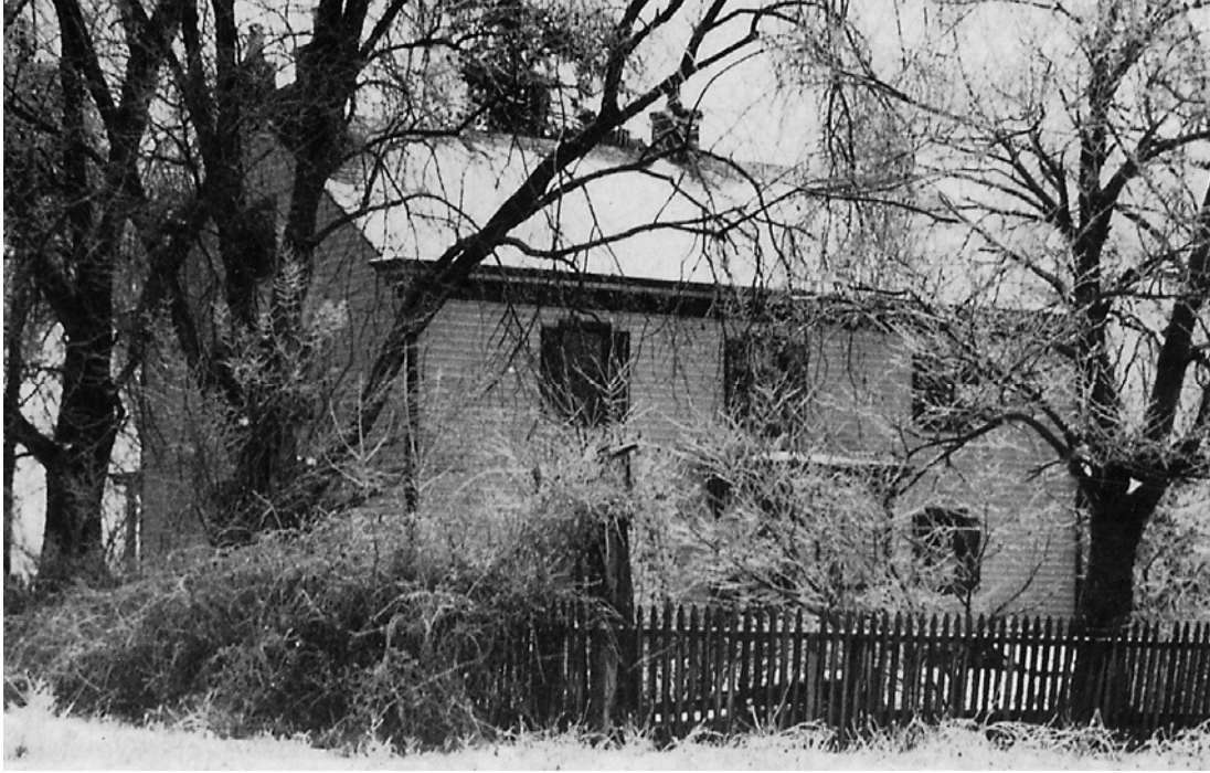
Photograph 17: Looking north at an early twentieth-century view of the rear of the main house showing the small central back porch and the symmetrical configuration of the windows. Note the wood drop siding.
