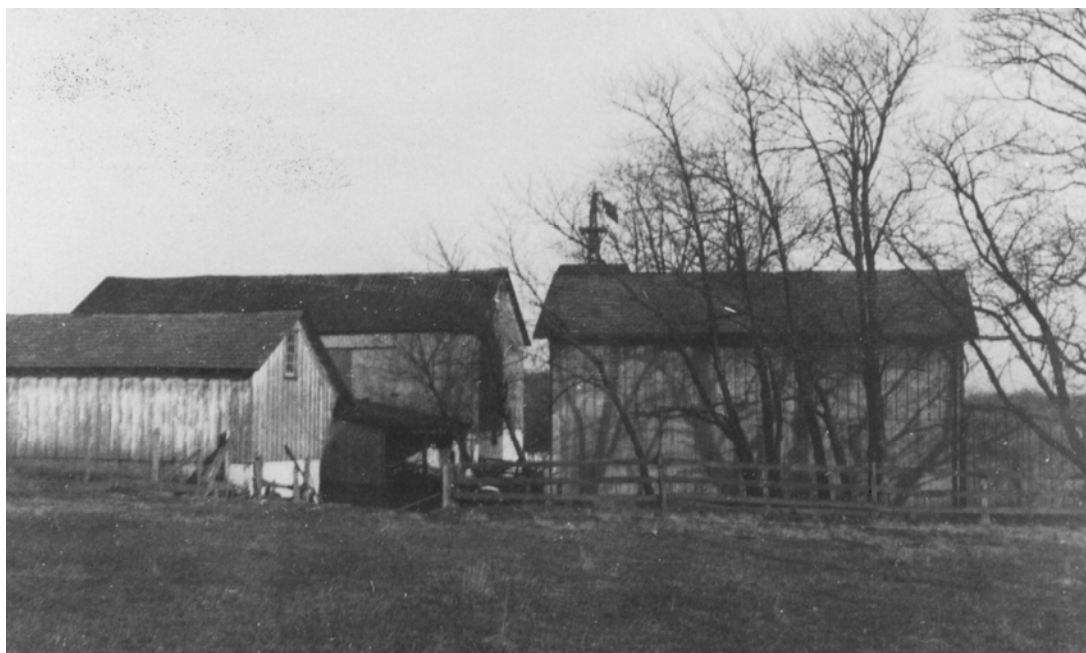
Photograph 21: Looking east toward the rear of the barn. Note the sliding doors to the threshing floor. An equipment shed is in the left foreground and the combination corn crib/wagon shed is to the right foreground.
