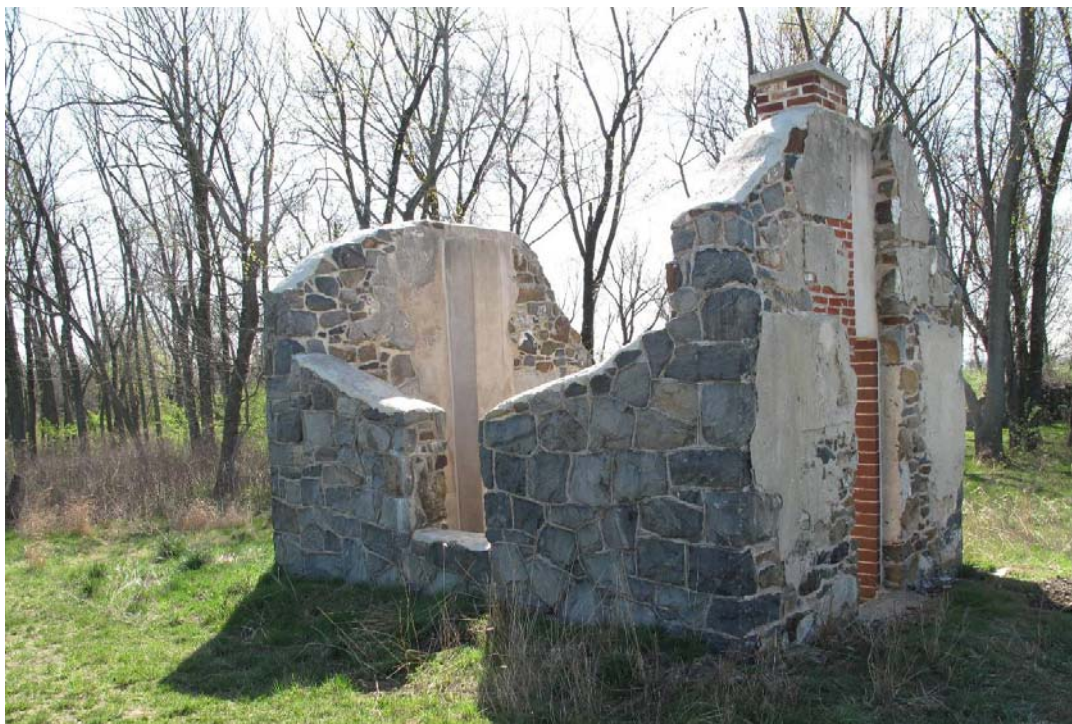
Photograph 20: Looking southwest at the milk house ruins after restoration by DeIDOT in the early 21 st century. Note the lines on the gable end where nailers would have supported a shed roof at this location.
