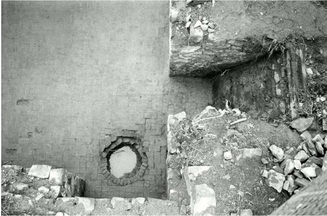
Photograph 39: View of the bulkhead at the southwest corner of the house foundation, facing east.
