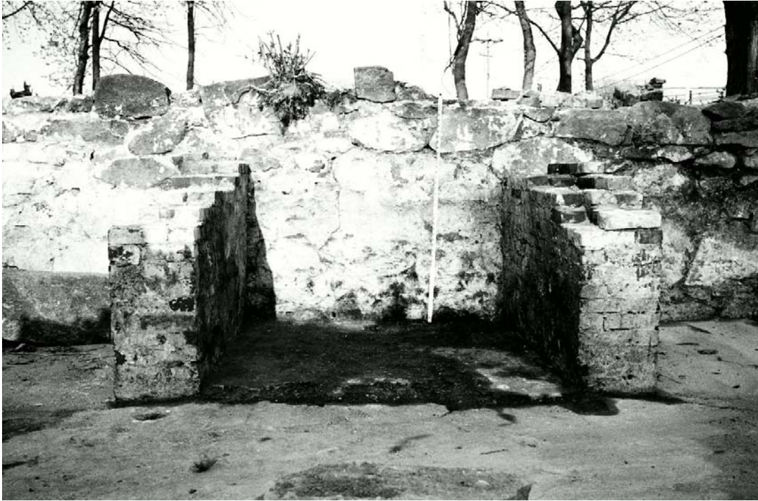
Photograph 30: Brick fireplace supports along the west wall of the east half of the cellar, facing west.
