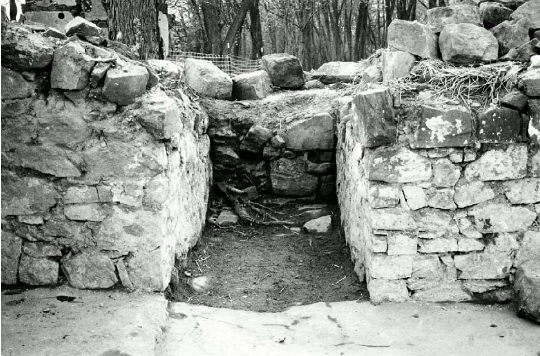
Photograph 28: Basement bulkhead at the southeast corner of the house, facing south.
