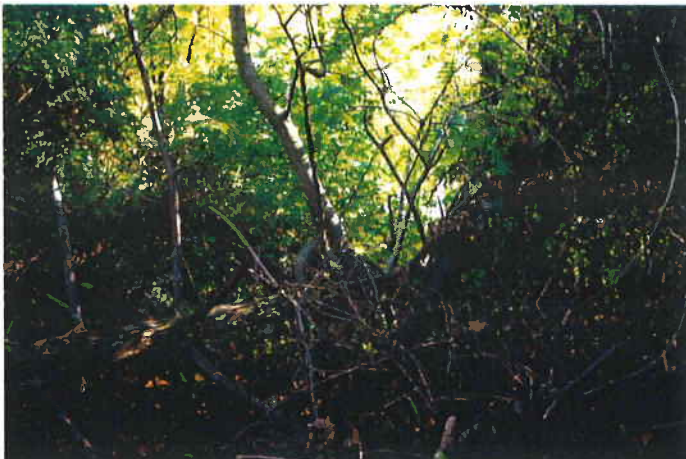
Photo 1 (See Figure 1 for location) Fallen white pine across Structure A.
