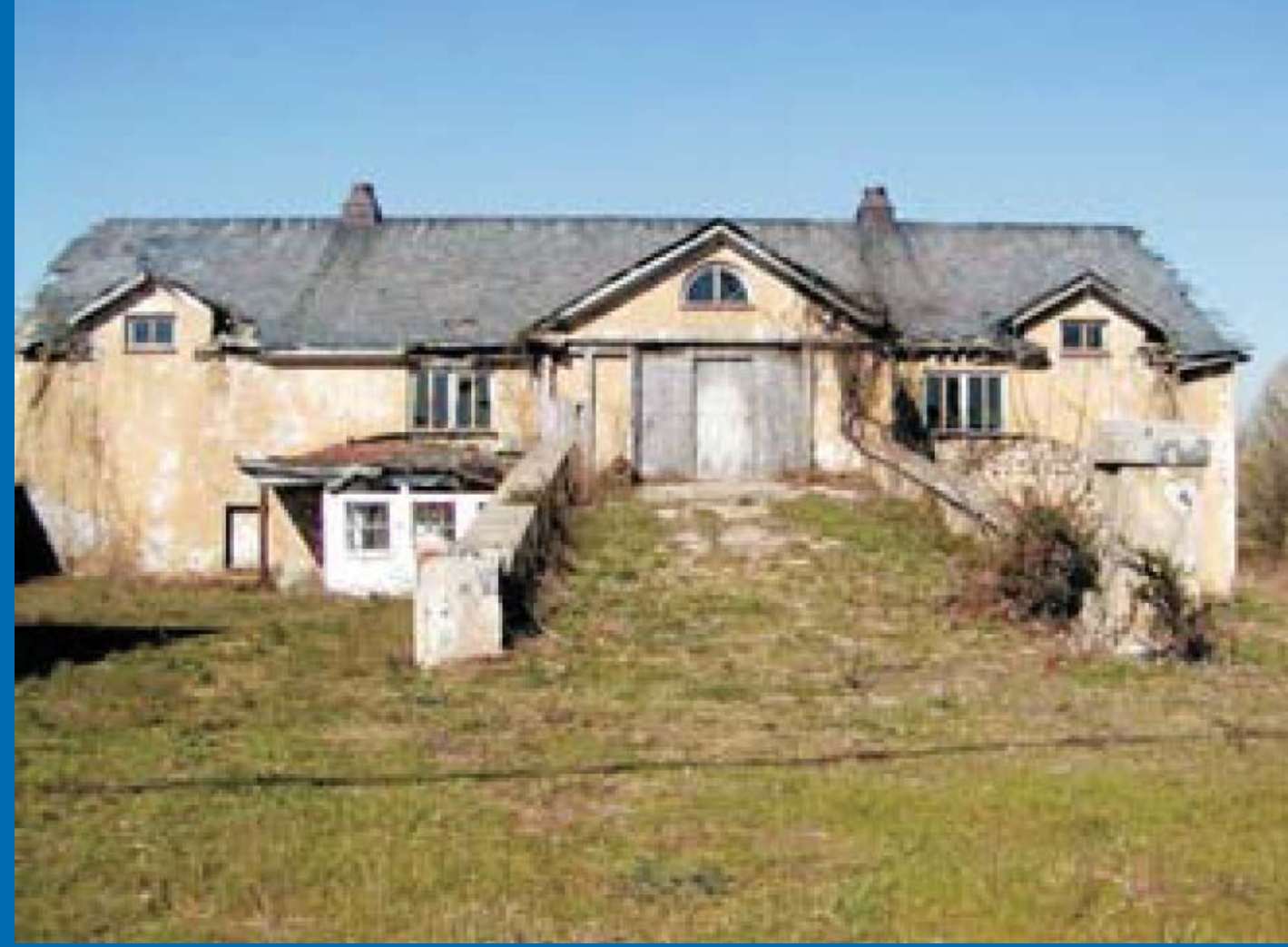
(below) View of Barn Before Renovations.
