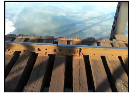
Figure 3. Typical Bolt Plate on Upper Shellpot Branch Rail Bridge
