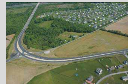
Sharp Curve South of Summit Bridge
