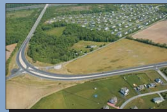
3 South of Summit Bridge Curve
