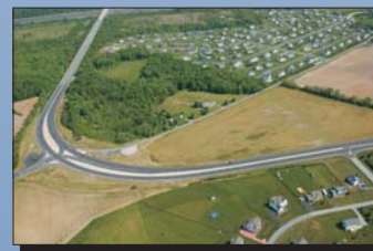
3 South of Summit Bridge Curve
