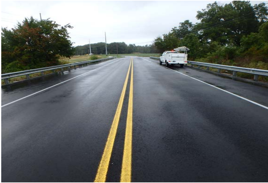
BR 2-066A Approach Roadway
