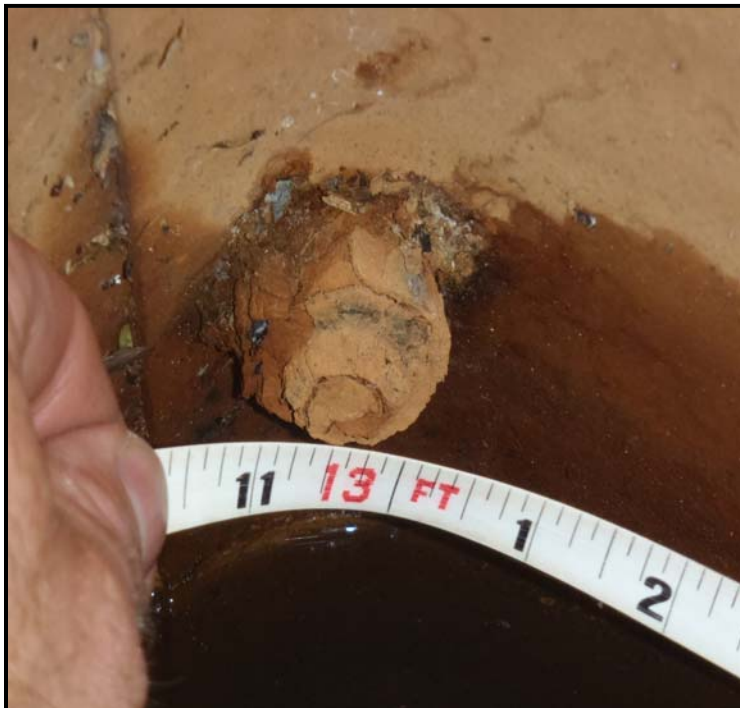
8. SPAN 2, E CELL, FASTENER SECTION LOSS AT 13 FEET FROM N END, LOOKING EAST
