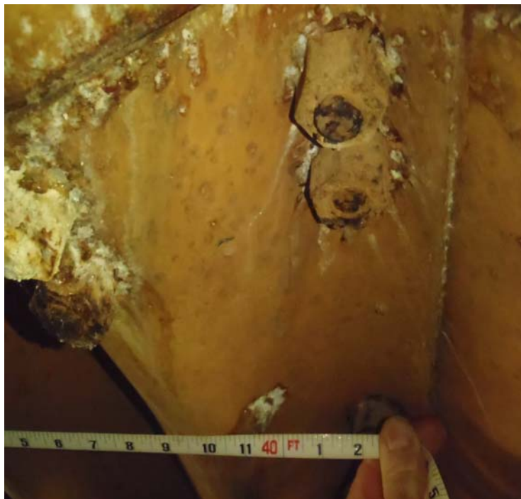
6. SPAN 1, W CELL, SMALL CORROSION BLISTERS & PITTING ON FASTENERS LOOK E
