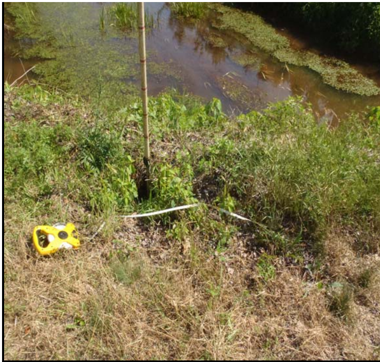
7. EROSION BETWEEN SPANS 1 & 2 IN THE NORTH SACK RIPRAP HEADWALL LOOK NORTH
