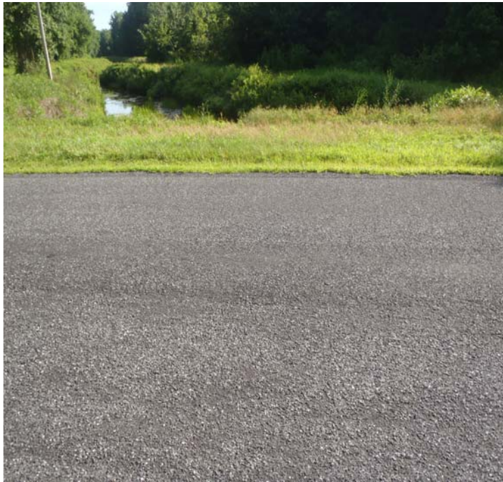
5. ASPHALT OVERLAY WEARING SURFACE LOOKING NORTH
